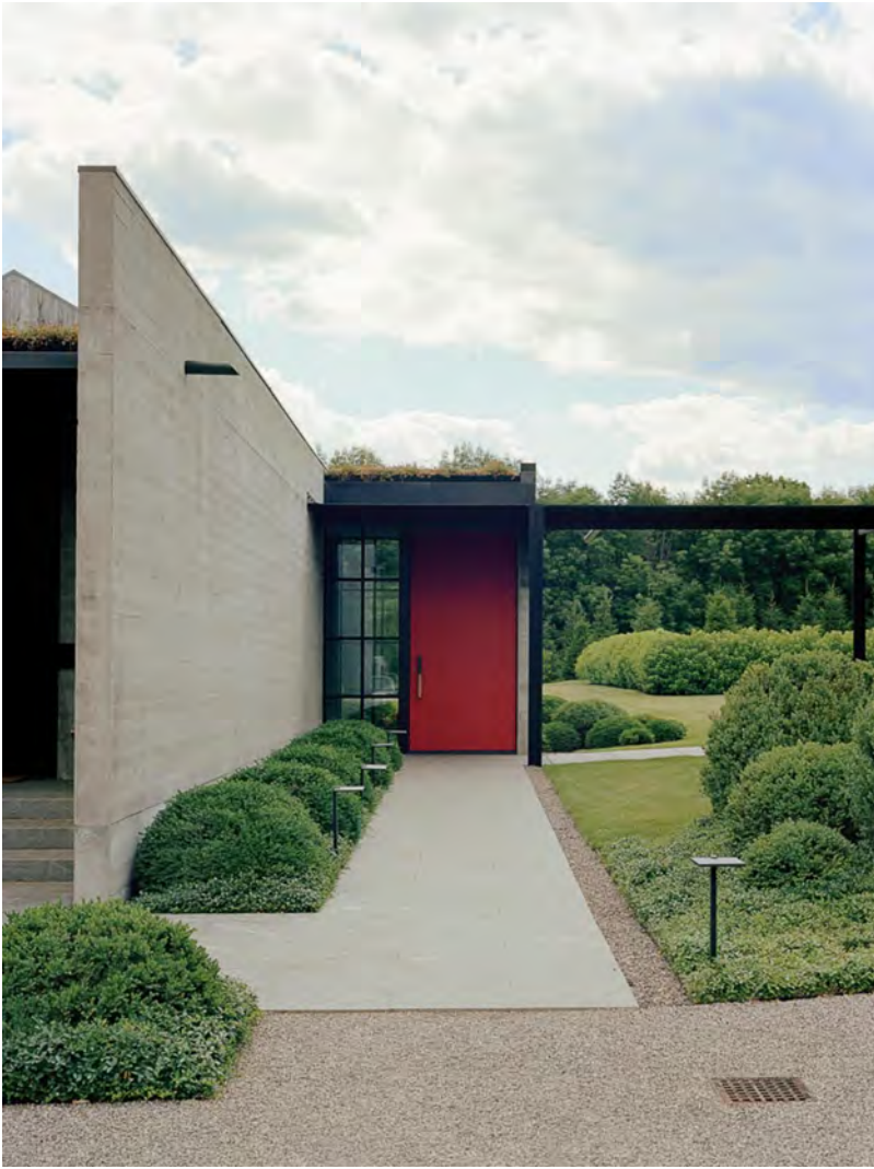
The carmine red of the massive steel front door was chosen from Le Corbusier's color palette. PHOTO: FRANÇOIS COQUEREL FOR WSJ. MAGAZINE
